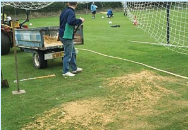
Once laid a light dressing should be applied along the joints
