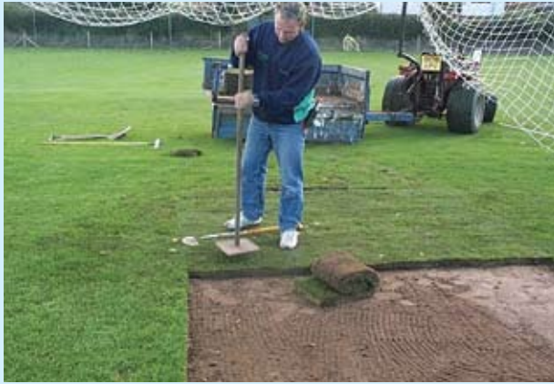
Turf should be tapped gently to level after laying
