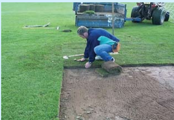
Turf should be laid in brick fashion to avoid drying out
