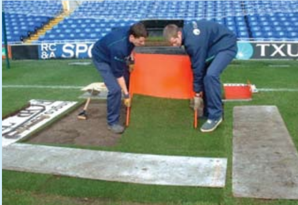
Slabs being laid. Note the boarding out of the existing goal area
